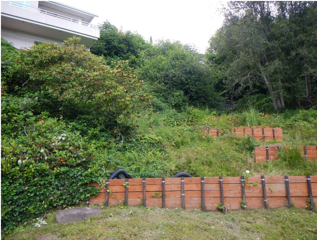
Timber catchment walls looking at west landslide.
