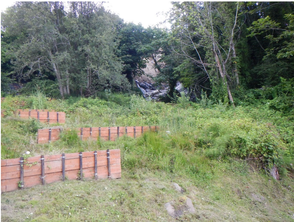
Timber catchment walls looking at east land slide.
